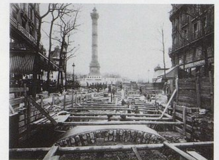
Construction of the First Metro Line: Work in Rue Saint-Antoine Archives de Paris
