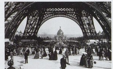
The Universal Exhibition of 1889. ND-Viollet Both the Palais du Trocadéro (the dome of which can be seen in the background) and the Eiffel Tower were built specially for the Universal Exhibition.
